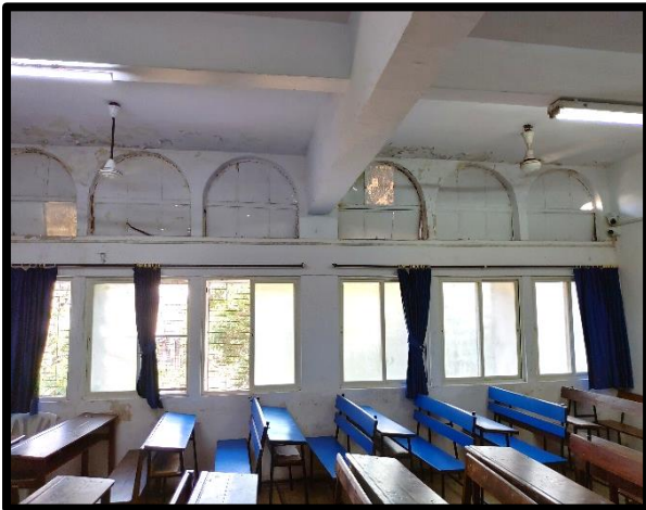
Good daylight and Ventilation in classrooms
